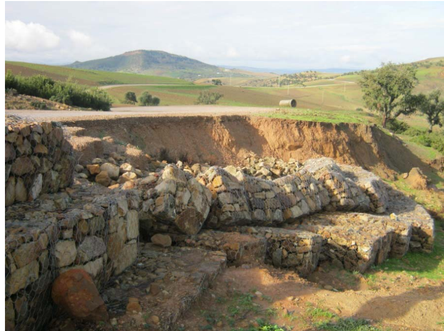
Photo 4: Reactivated old landslide
